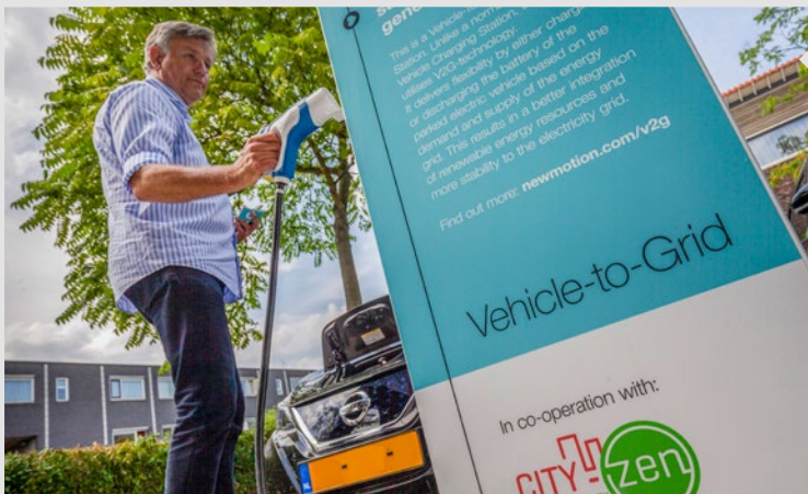
A man connects his electric car to a public charging pole, part of the City-zen smart city project in Amsterdam, the Netherlands, which received funding from the EU's Horizon 2020 programme. This funding forms part of President Juncker's Investment Plan for Europe, which surpassed its original €315 billion target for investment on 18 July 2018.
